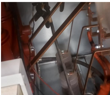
Carrying out of Breaker contact resistance in progress.
