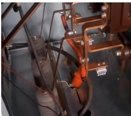
Cleaned Panel after maintenance.
