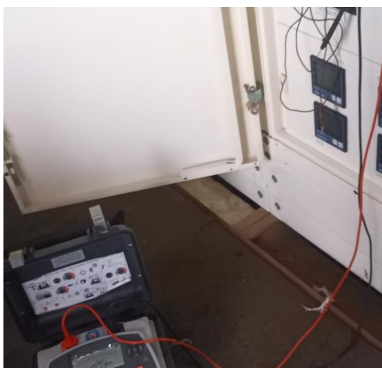
Carrying of LV B/B Insulation Resistance Test.
