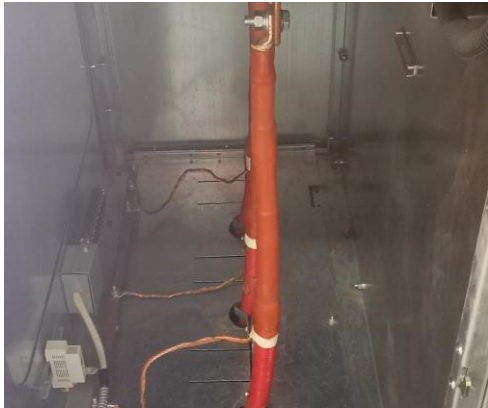
Interior panel after maintenance
