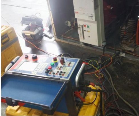
Testing of contact resistance of breaker using CPC100
