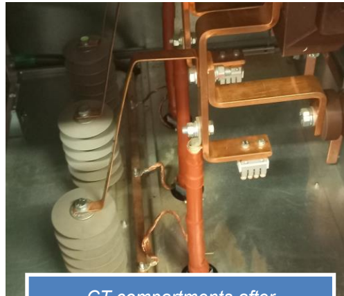
CT compartments after maintenance.
