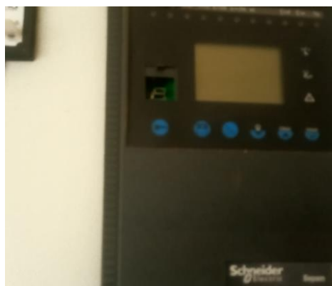
Schneider Electric/Sepam relay black out.
