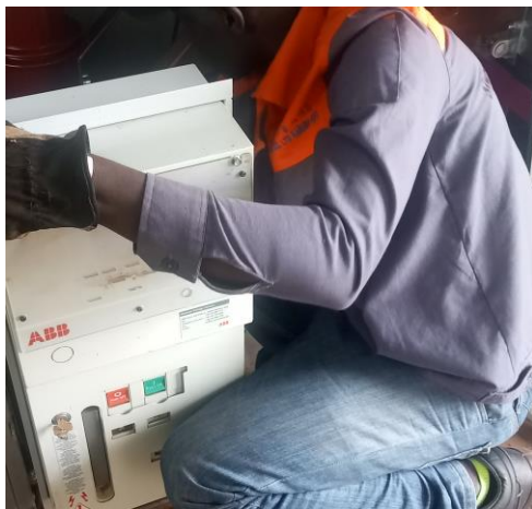
Maintenance and terminations checkups ongoing
