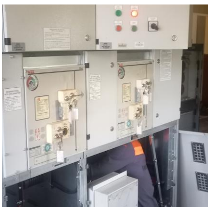
Checking terminations and Vacuum cleaning ongoing.
