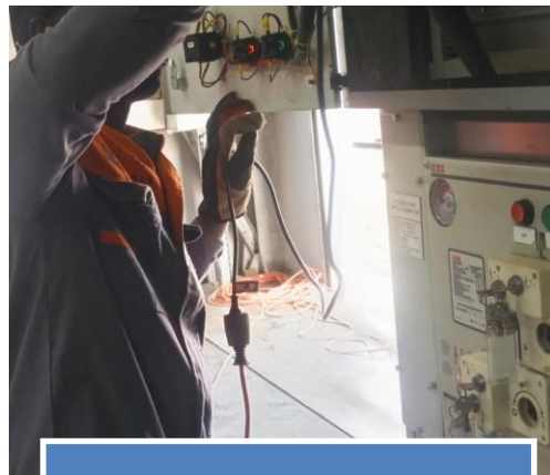
Checking control wiring terminations
