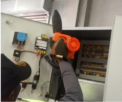
Vacuum cleaning of control panel.
